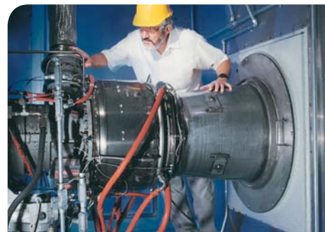
The bulk of engine maintenance can be performed on-site.
