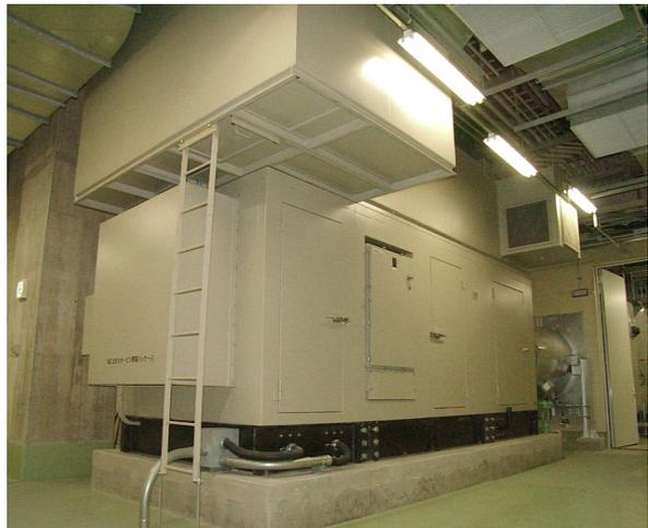
The ASE40 gas turbine is used to offset expensive grid power and to convert wasteful heat to useful energy for chilling and heating applications.
