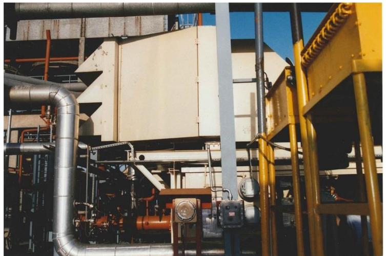
The ASE40 gas turbine drives a centrifugal gas compressor on a continuous duty basis.
