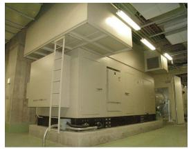
The ASE40 gas turbine is used to offset expensive grid power and convert wasteful heat to useful energy for chilling and heating applications.
