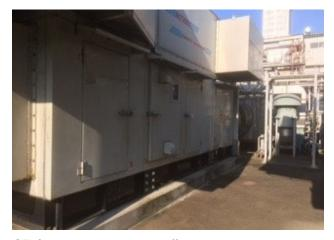
The ASE50 gas turbine is used to offset expensive grid power and convert wasteful heat to useful steam for a beverage processing plant.
